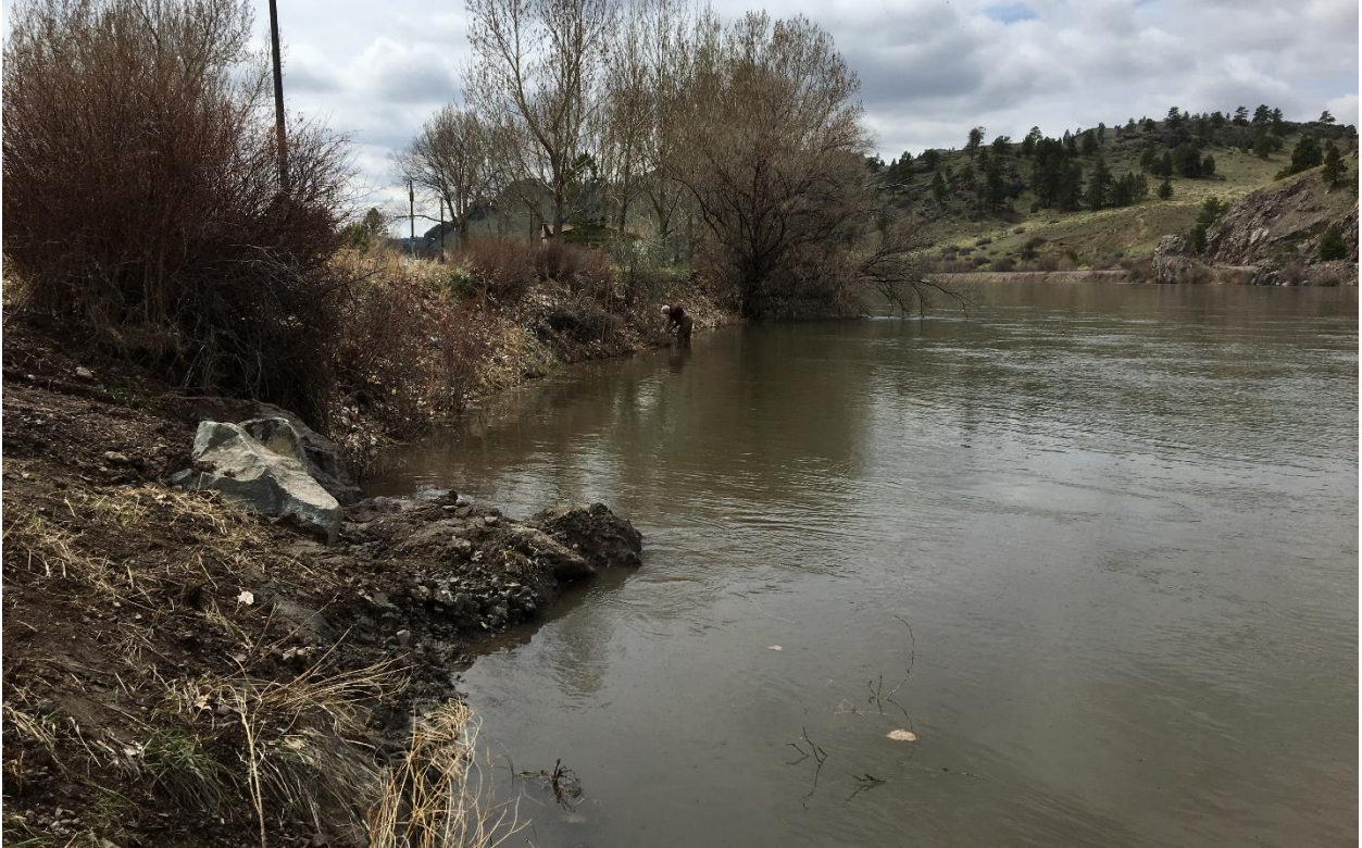
Photo 2. Looking upstream. After bank work. Photo taken during high water. Most of the added rocks are submerged. April 2018.
