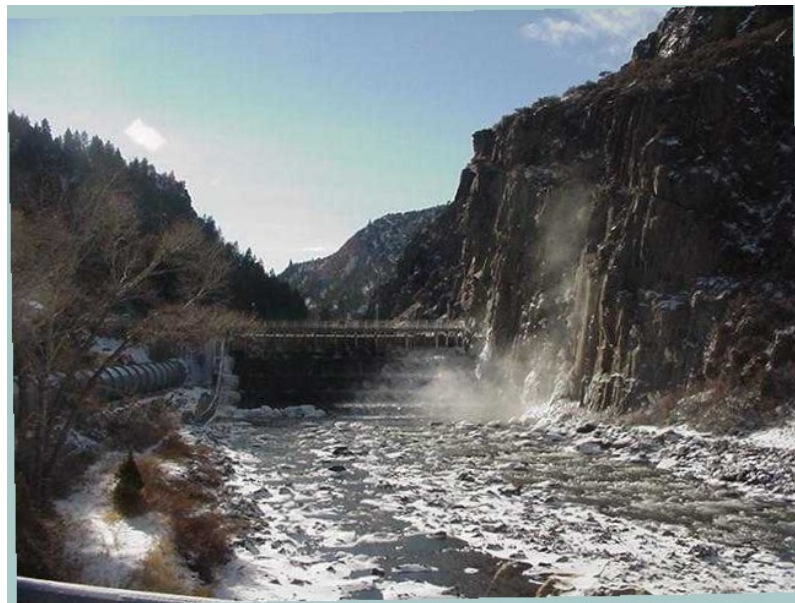
Figure 6. Ennis Dam on the Madison River. The gray metal pipeline (penstock) on the left transports water from Ennis Reservoir to the Madison Powerplant, approximately 1.4 miles downstream from the dam.
