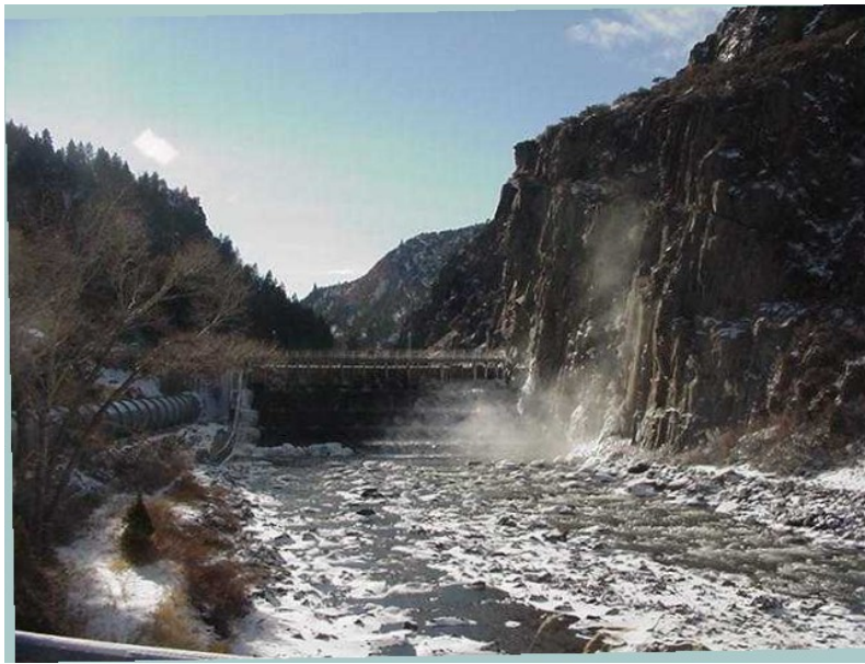
Figure 6. Ennis Dam on the Madison River. The gray metal pipeline (penstock) on the left transports water from Ennis Reservoir to the Madison Powerplant, approximately 1.4 miles downstream from the dam.
