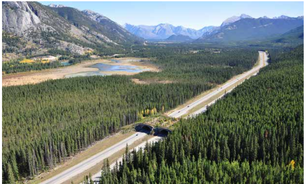
Aerial view of the Trans-Canada Highway overpass wildlife crossing between Banff and Lake Louise, Alberta.
