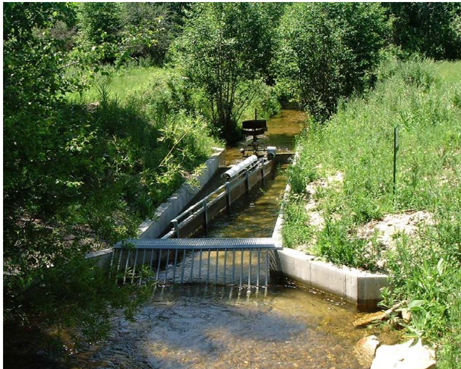
Figure 36. Self-cleaning fish screen.
