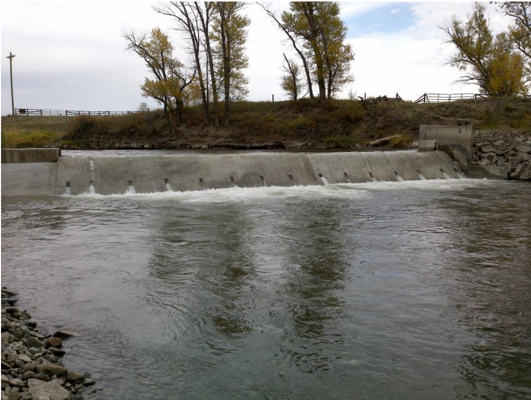
Figure 4: Chadbourne Diversion in 2013 after repair and retrofit to act as a fish barrier.
