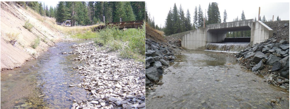
Figure 6: Before (left) and after (right) photos of the fish passage barrier at Crandall Creek Campground. Photos courtesy of the Custer Gallatin National Forest.
