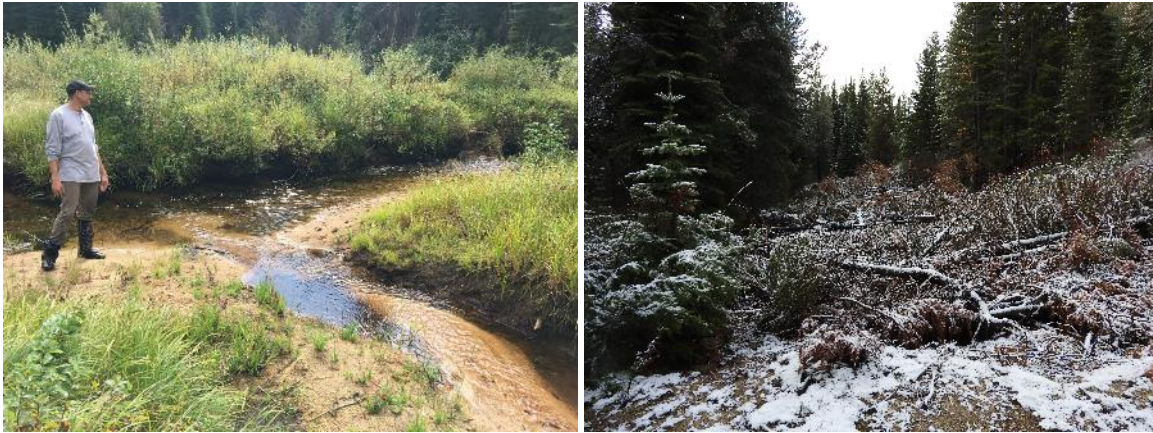
FIGURE 20. WEST FORK OF LOLO CREEK AND LEE CREEK BEFORE RESTORATION (L) AND AFTER (R) ROADS WERE DECOMMISSIONED. BEFORE PHOTO COURTESY OF CLARK FORK COALITION.
