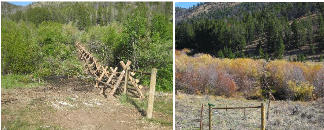
FIGURE 85. JOHNSON CREEK FENCE AFTER CONSTRUCTION (L; 2014) AND IN 2020 (R). THE FENCE AND RIPARIAN AREA REMAINS INTACT.
