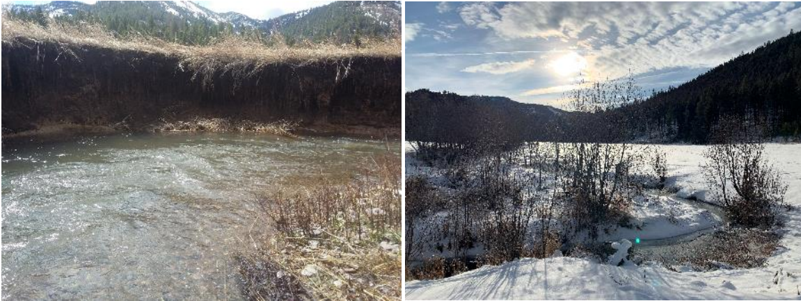
FIGURE 13. MILLER CREEK BEFORE (L) AND AFTER (R) CHANNEL RECONSTRUCTION AND REVEGETATION. BEFORE PHOTO COURTESY OF CLARK FORK COALITION.
