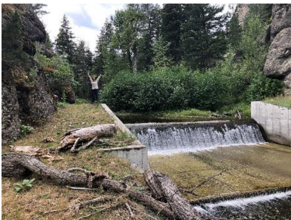
FIGURE 56. LOWER DEER CREEK BARRIER FRONT VIEW. LOGS WERE DEPOSITED ON WINGWALLS DURING FLOODING IN 2011.
