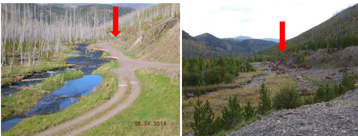
FIGURE 25. COPPER CREEK BEFORE RESTORATION (L), WITH THE STREAM ERODING THE ROAD. THE ROAD WAS MOVED TO THE SIDESLOPE AND OUT OF THE FLOODPLAIN (R). RED ARROWS DENOTE COMMON FEATURES. BEFORE PHOTO COURTESY OF BIG BLACKFOOT CHAPTER OF TROUT UNLIMITED.
