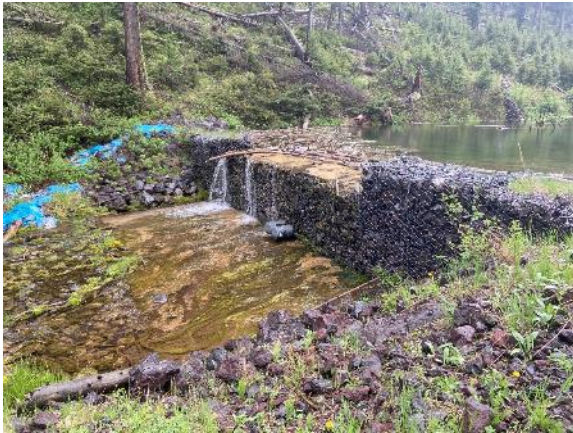
FIGURE 48. THE LAKE CREEK FISH BARRIER ON JUNE 6, 2020.
