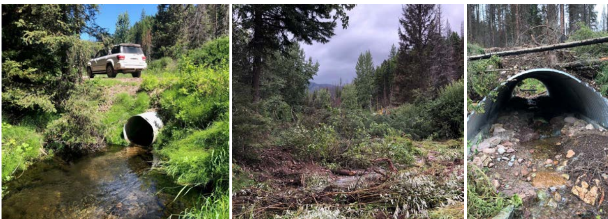
FIGURE 26. COTTONWOOD CREEK AND NORTH FORK COTTONWOOD CREEK. BEFORE RESTORATION, AN UNDERSIZED CULVERT IMPEDED FISH PASSAGE (L). THE ROAD WAS DECOMMISSIONED AND REROUTED (CENTER), AND A NEW CULVERT WAS INSTALLED (R). PHOTOS COURTESY OF BIG BLACKFOOT CHAPTER OF TROUT UNLIMITED.
