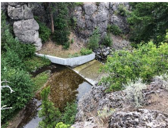
FIGURE 55. VIEW OF THE LOWER DEER CREEK BARRIER FROM TOP OF CANYON.
