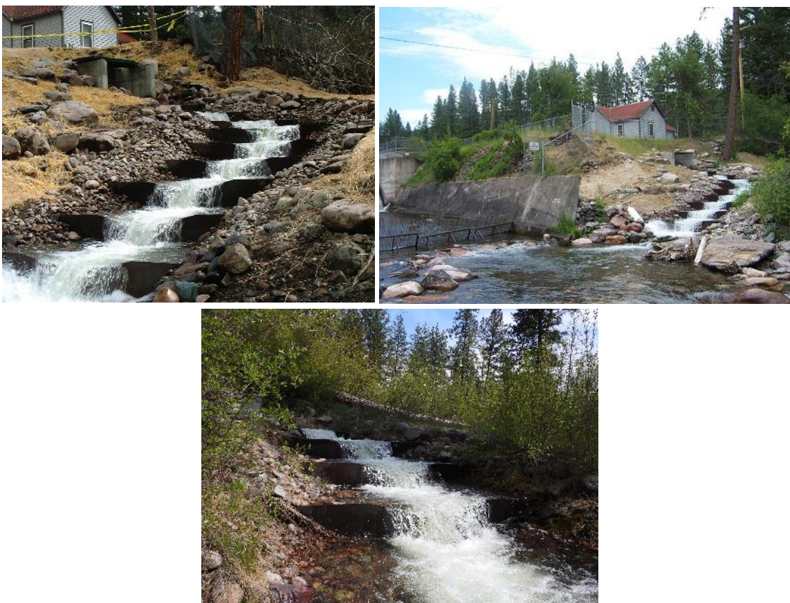
FIGURE 98. RATTLESNAKE CREEK FISH LADDER AFTER CONSTRUCTION (TOP LEFT; 2003), IN 2014 (TOP RIGHT) AND IN 2020 (BOTTOM). THE FISH LADDER WAS REMOVED IN 2020 WITH THE REMOVAL OF RATTLESNAKE DAM.
