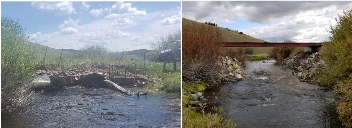
FIGURE 9. ROSS FORK ROCK CREEK BEFORE (L) AND AFTER (R) THE PROJECT; REPLACING UNDERSIZED CULVERTS WITH A RAIL CAR FARM BRIDGE. PHOTOS COURTESY OF TROUT UNLIMITED.
