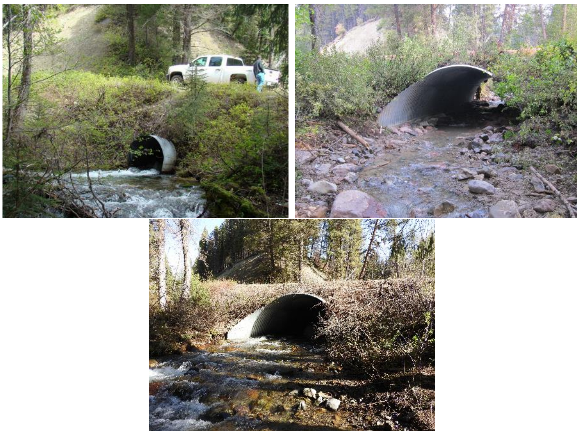
FIGURE 109. YUKON CREEK FISH PASSAGE BEFORE CONSTRUCTION (TOP LEFT), AFTER CONSTRUCTION (TOP RIGHT; 2015), AND IN 2019 (BOTTOM).
