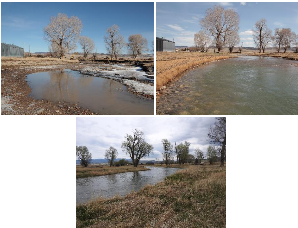
FIGURE 102. RUBY RIVER CHANNEL BEFORE CONSTRUCTION (TOP LEFT), AFTER CONSTRUCTION (TOP RIGHT; 2015), AND IN 2019 (BOTTOM).
