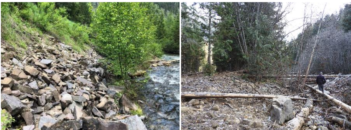
FIGURE 24. CEDAR CREEK BEFORE RESTORATION (L), WITH RIP RAP ALONG THE CREEK. AFTER (R) RESTORATION, WITH THE ROAD RELOCATED AND INSTREAM FISH HABITAT ADDED. BEFORE PHOTO BY TROUT UNLIMITED.
