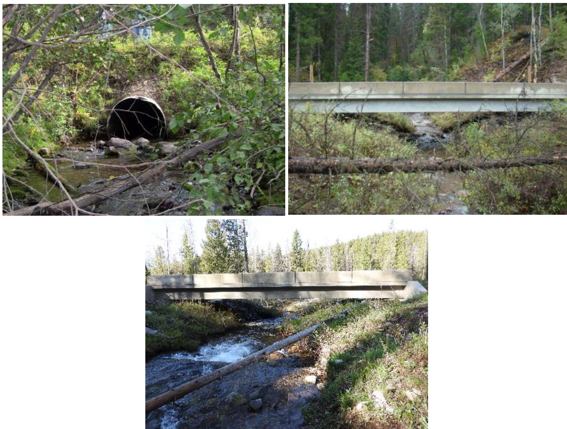
FIGURE 87. KLONDIKE CREEK CULVERT TO BRIDGE PROJECT BEFORE (TOP LEFT), AFTER (TOP RIGHT; 2013), AND IN 2019 (BOTTOM).
