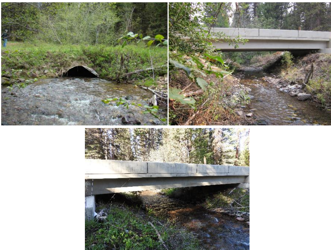
FIGURE 106. THEODORE CREEK BEFORE THE BRIDGE WAS INSTALLED (TOP LEFT), AFTER CONSTRUCTION (TOP RIGHT; 2015) AND 2019 (BOTTOM).
