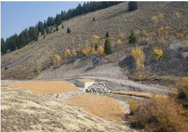
FIGURE 10. SELWAY CREEK BARRIER AFTER CONSTRUCTION.
