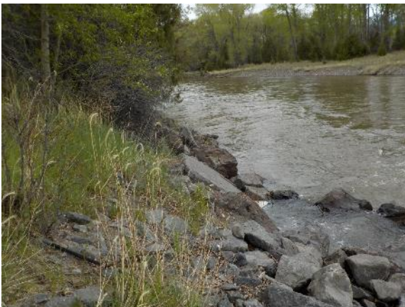
FIGURE 74. BANK ARMORING IN THE PROJECT AREA.
