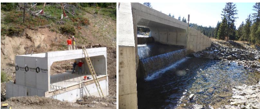
FIGURE 103. SHIELDS RIVER BARRIER BEING INSTALLED (L) AND AFTER CONSTRUCTION (R; 2019).
