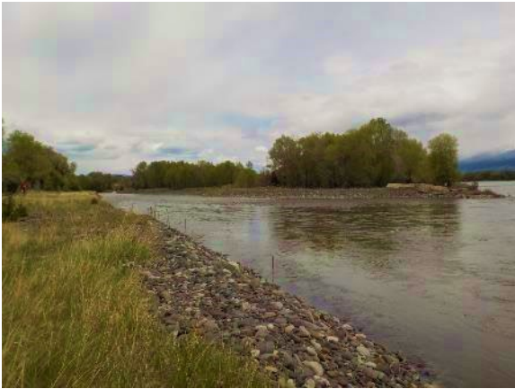
FIGURE 71. TRAPEZOIDAL CHANNEL GEOMETRY, COBBLE BANKS, AND JERSEY BARRIERS ABANDONED ON THE UPSTREAM END OF MID-CHANNEL BAR.
