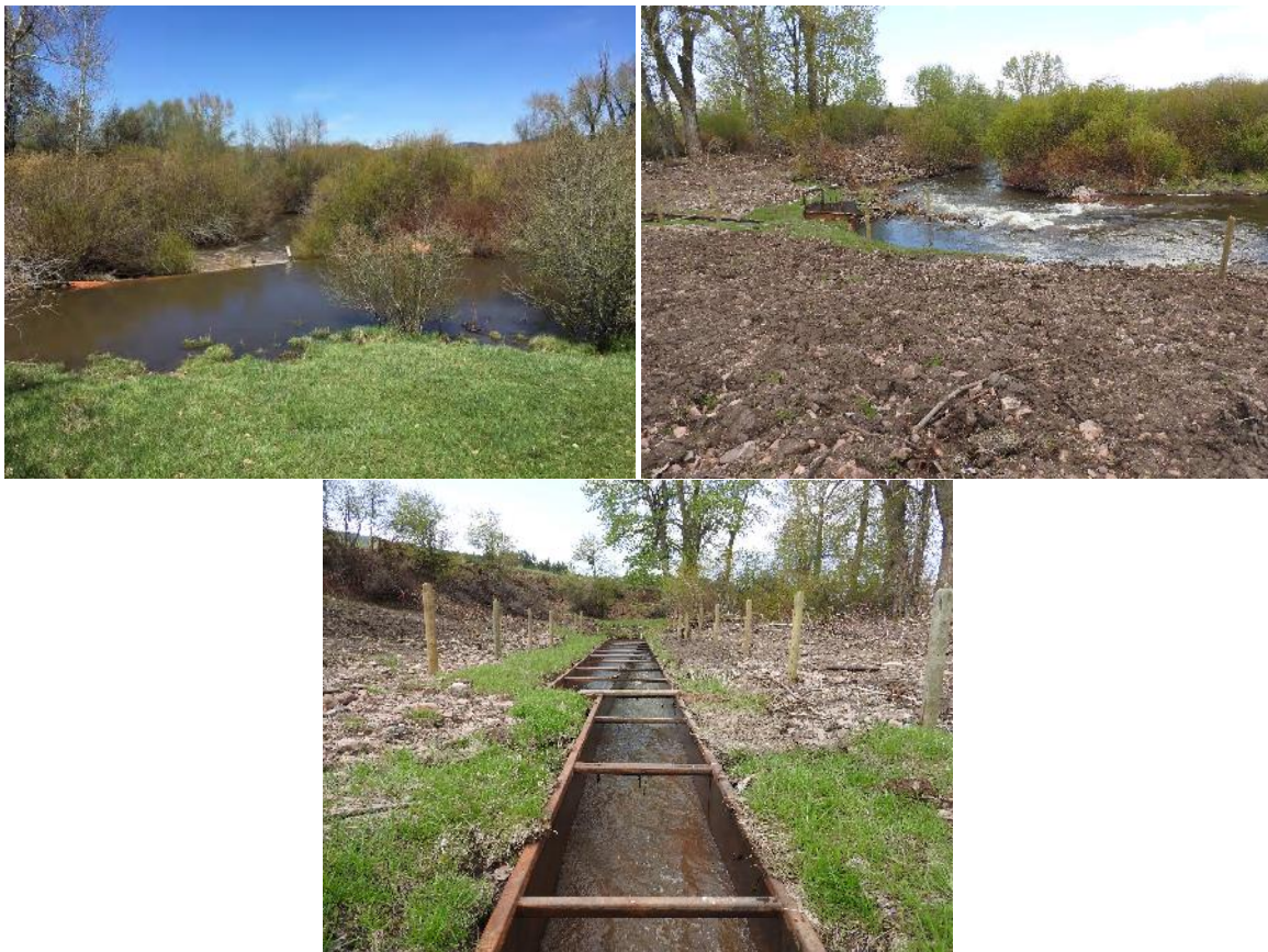
FIGURE 36. NEVADA CREEK DIVERSION BEFORE (TOP L) CONSTRUCTION. THE IRRIGATION DIVERSION WAS UPGRADED (TOP R) AND A FISH SCREEN WAS INSTALLED (BOTTOM) BEHIND THE HEADGATE. BEFORE PHOTO COURTESY OF BIG BLACKFOOT CHAPTER OF TROUT UNLIMITED.
