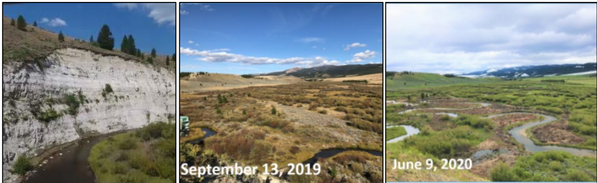
FIGURE 11. FRENCH CREEK CHANNEL RECONSTRUCTION BEFORE (L AND CENTER) AND AFTER (R). THE STREAM CHANNEL WAS MOVED AWAY FROM THE HIGHLY EROSIVE HILLSIDE (L PICTURE). PHOTOS COURTESY OF BIG HOLE WATERSHED COMMITTEE.
