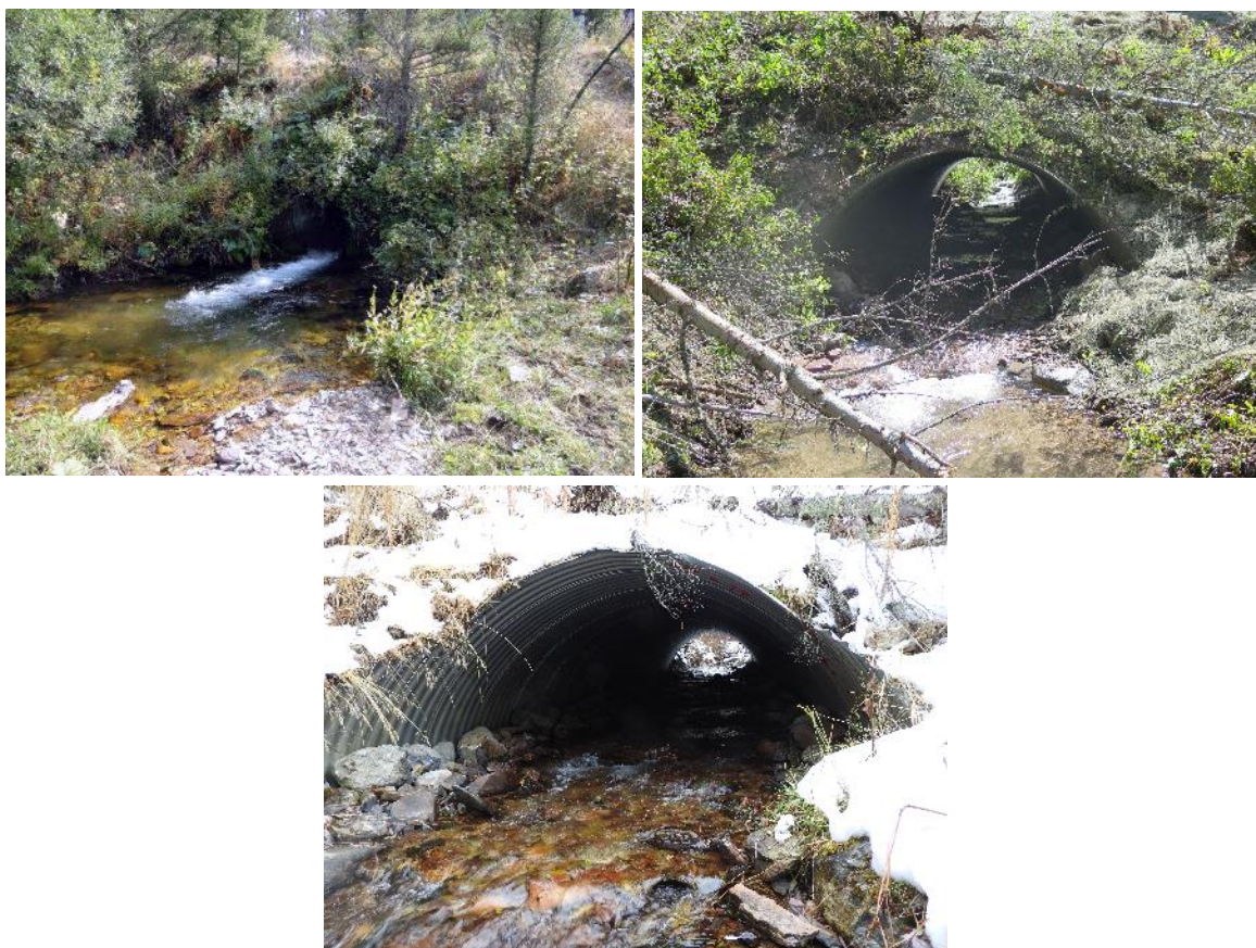
FIGURE 86. GLEASON CREEK FISH PASSAGE PROJECT BEFORE (TOP LEFT), AFTER (TOP RIGHT; 2014), AND IN 2020 (BOTTOM).
