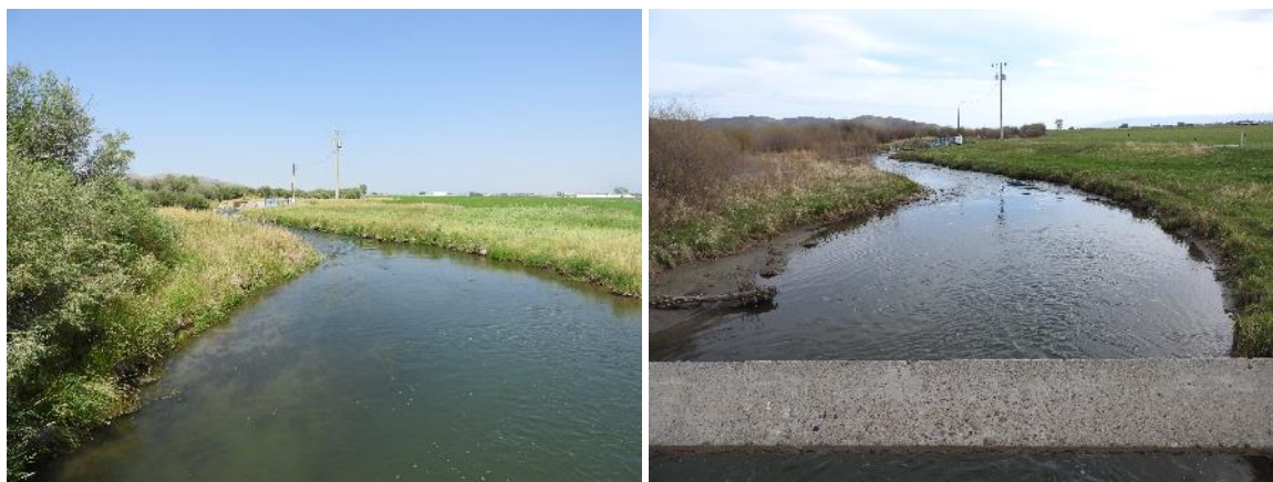
FIGURE 93. POINDEXTER SLOUGH AFTER CONSTRUCTION (L; 2016) AND IN 2019 (R).
