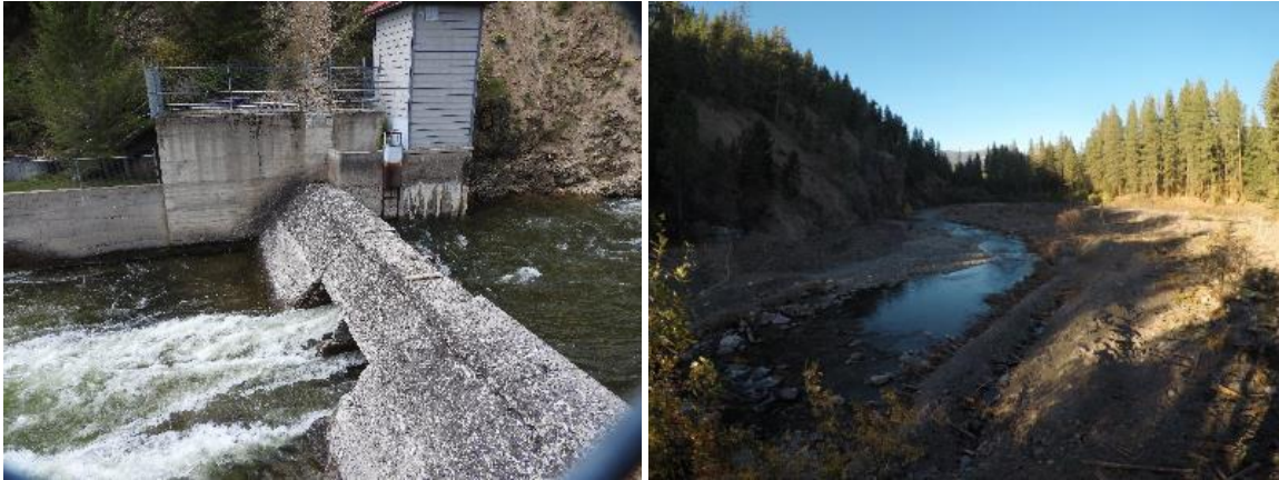
FIGURE 8. RATTLESNAKE CREEK BEFORE (L) AND AFTER (R) DAM REMOVAL. THE FORMER DAM SITE IS IN THE BOTTOM LEFT AREA OF THE AFTER PHOTO. AFTER PHOTO COURTESY OF MONTANA TROUT UNLIMITED.
