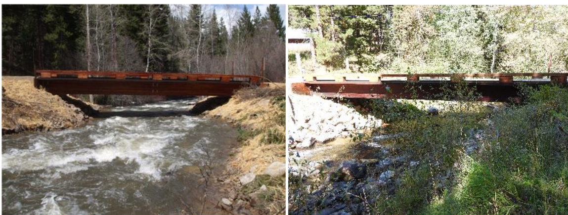
FIGURE 107. WARM SPRINGS BRIDGE AFTER CONSTRUCTION (L; 2011) AND IN 2020 (R).
