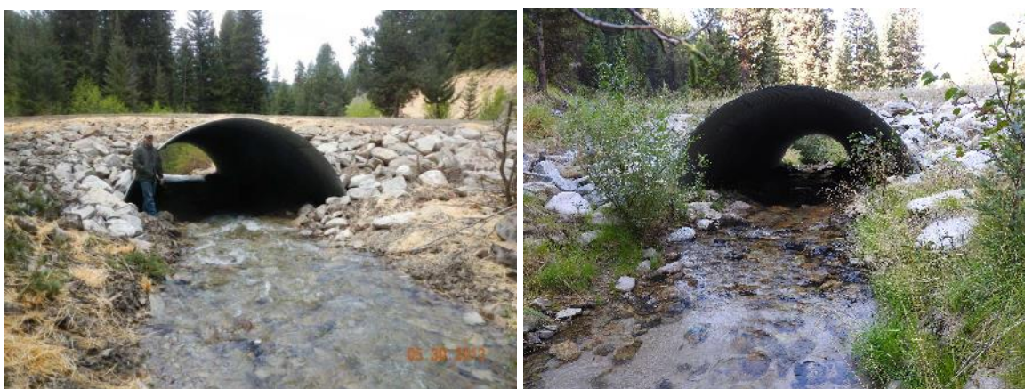
FIGURE 89. LITTLE BOULDER CREEK AFTER CONSTRUCTION (L; 2013) AND IN 2020 (R).
