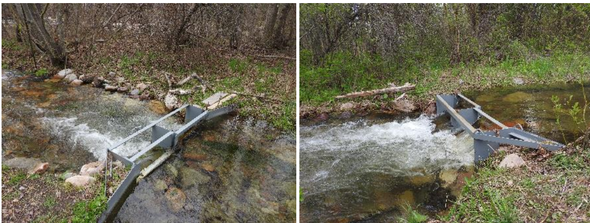
FIGURE 99. RATTLESNAKE CREEK FISH SCREEN AFTER CONSTRUCTION (L; 2015) AND IN 2020 (R).
