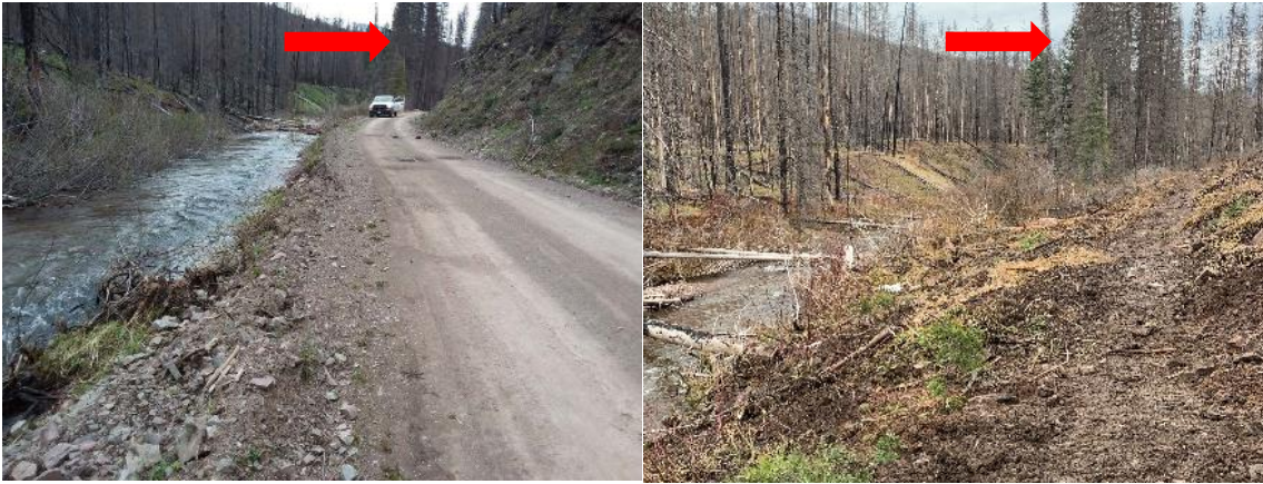
FIGURE 14. MORELL CREEK ROAD BEFORE (L) AND AFTER (R) DECOMMISSIONING. BEFORE PHOTO COURTESY OF BIG BLACKFOOT CHAPTER TROUT UNLIMITED. RED ARROWS DENOTE THE SAME TREES IN EACH PHOTO.
