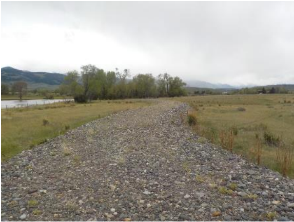
FIGURE 73. ELEVATED ROADBED MADE FROM SPOILS FROM YEARS OF DREDGING IN THE PROJECT AREA.
