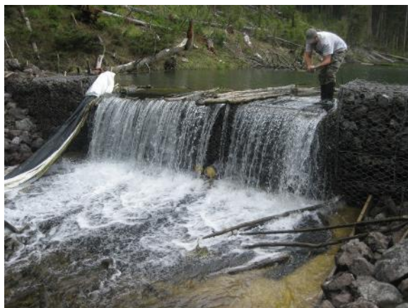
FIGURE 47. LAKE CREEK FISH BARRIER ONE YEAR AFTER CONSTRUCTION.
