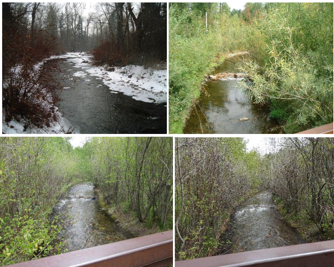
FIGURE 97. RATTLESNAKE CREEK CHANNEL RESTORATION BEFORE CONSTRUCTION (TOP LEFT), AFTER CONSTRUCTION (TOP RIGHT; 2009), 2015 (BOTTOM LEFT), AND IN 2020 (BOTTOM RIGHT).
