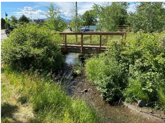
FIGURE 63. FOOTBRIDGE OVER A RESTORED SECTION OF MANDEVILLE CREEK SHOWING A RIFFLE/POOL SEQUENCE.
