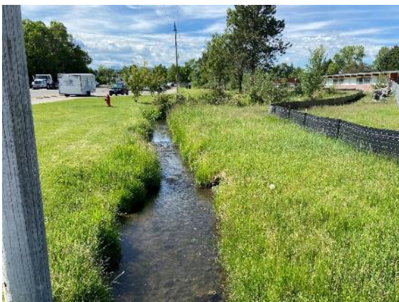
FIGURE 65. LOWER, UNRESTORED REACH OF MANDEVILLE CREEK ON THE BOZEMAN HIGH SCHOOL CAMPUS.
