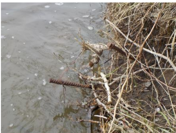
FIGURE 75. REBAR USED TO ANCHOR WILLOW/ALDER BUNDLES INTO BANKS.
