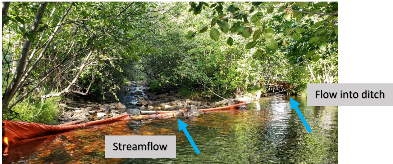
Looking downstream at the tarp and pole diversion in the stream. Ditch begins on right bank.
