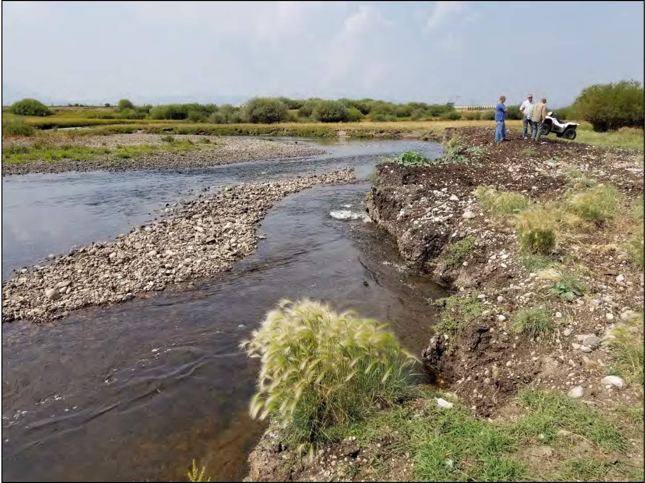
Streambank 1 prior to temporary fix.
