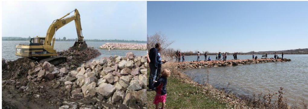
Figure 2. Examples of rock jetties; $104.50 per foot (~$15,675 for rock in one jetty)
