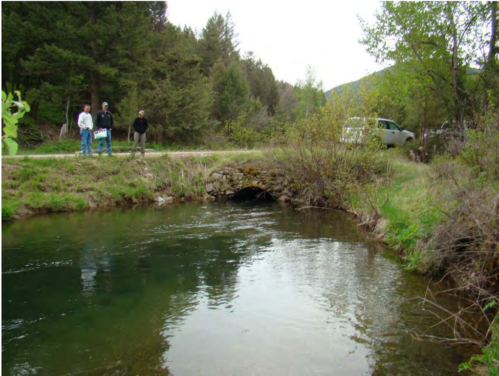
Existing Culvert on Poorman Creek Stemple Pass Rd Mile 5.8
