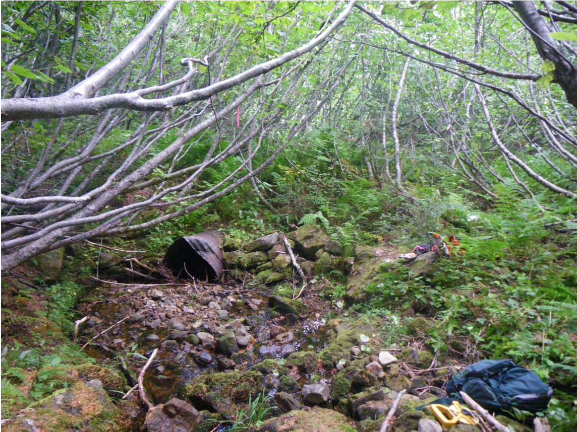
Station 202+50 Perennial stream - undersized culvert failing, shows signs of overtopping, washout risk
