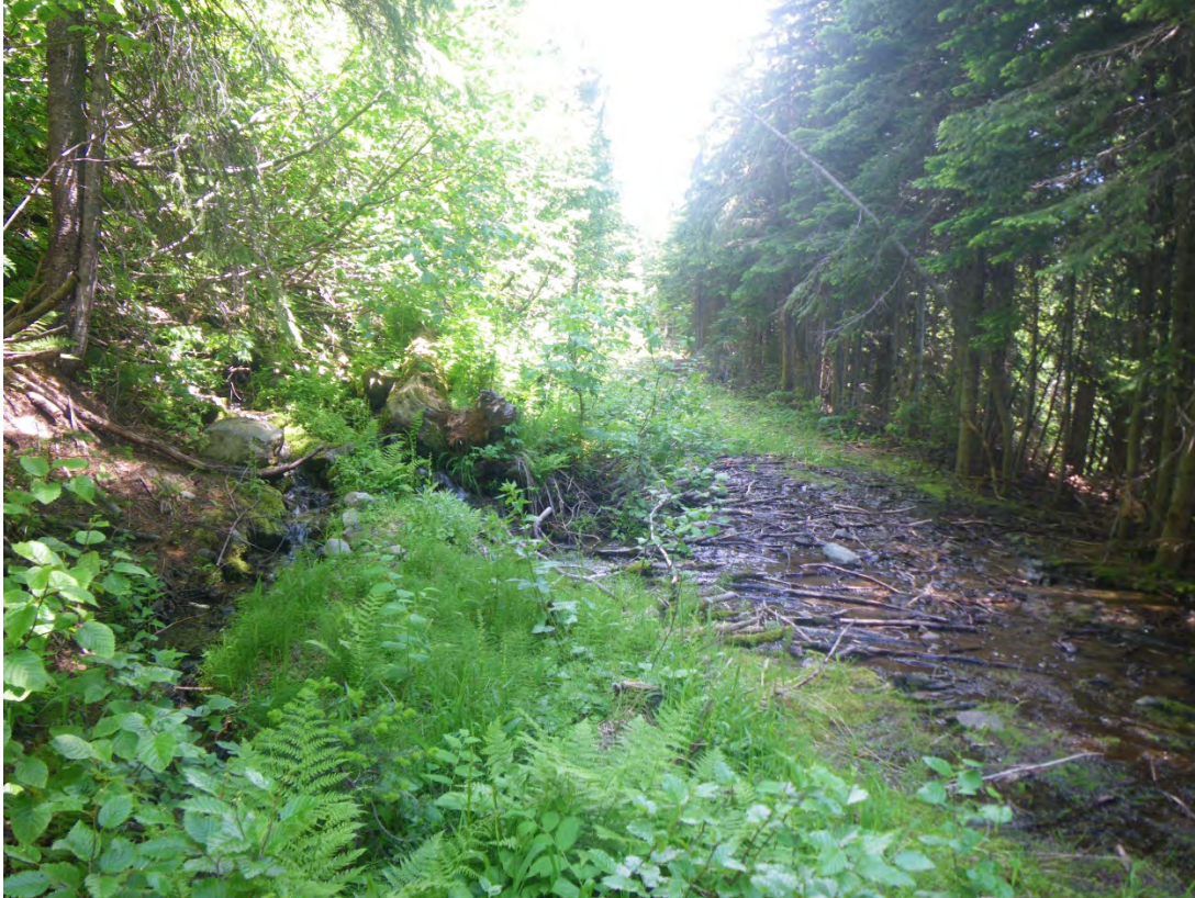
Station 37+20 Perennial stream/slide and saturated roadbed, slide risk
