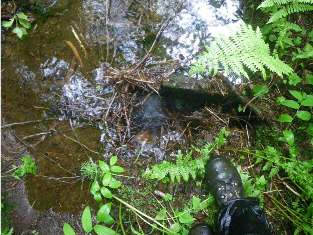
Station 8+50 Failing wooden culvert on perennial stream, washout risk
