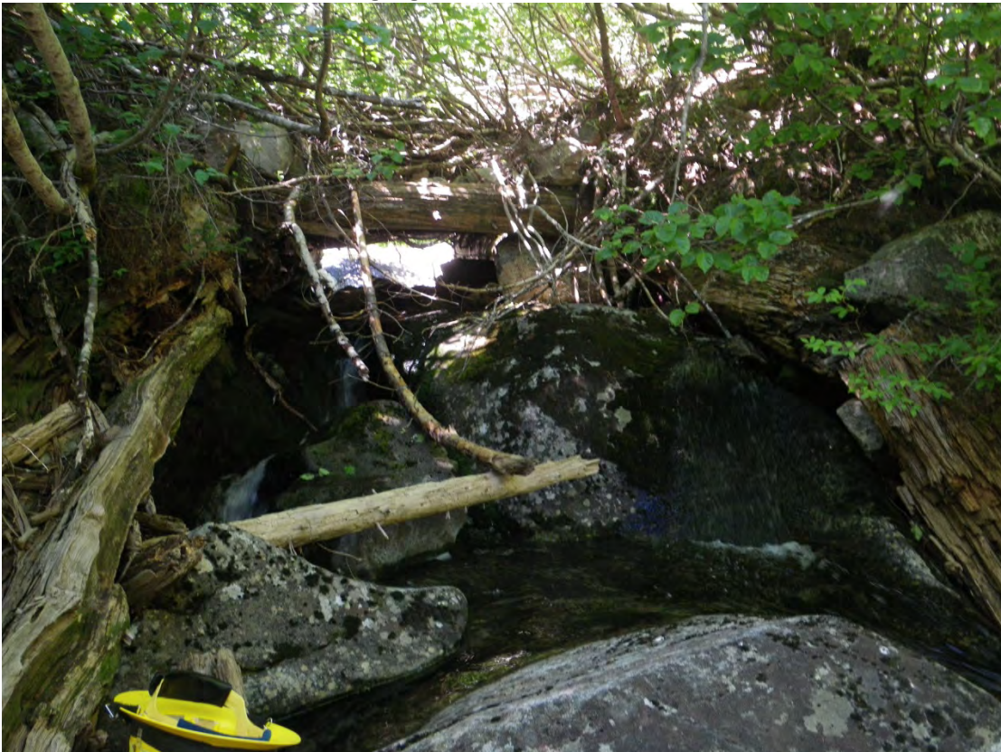
Station 17+48 Hidden Creek failing log/earth structure, channel restriction
