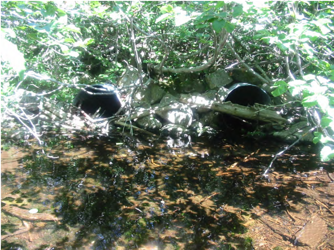
Station 90+70 –Hidden Creek tributary, undersized culverts show signs of plugging & overtopping, washout risk
