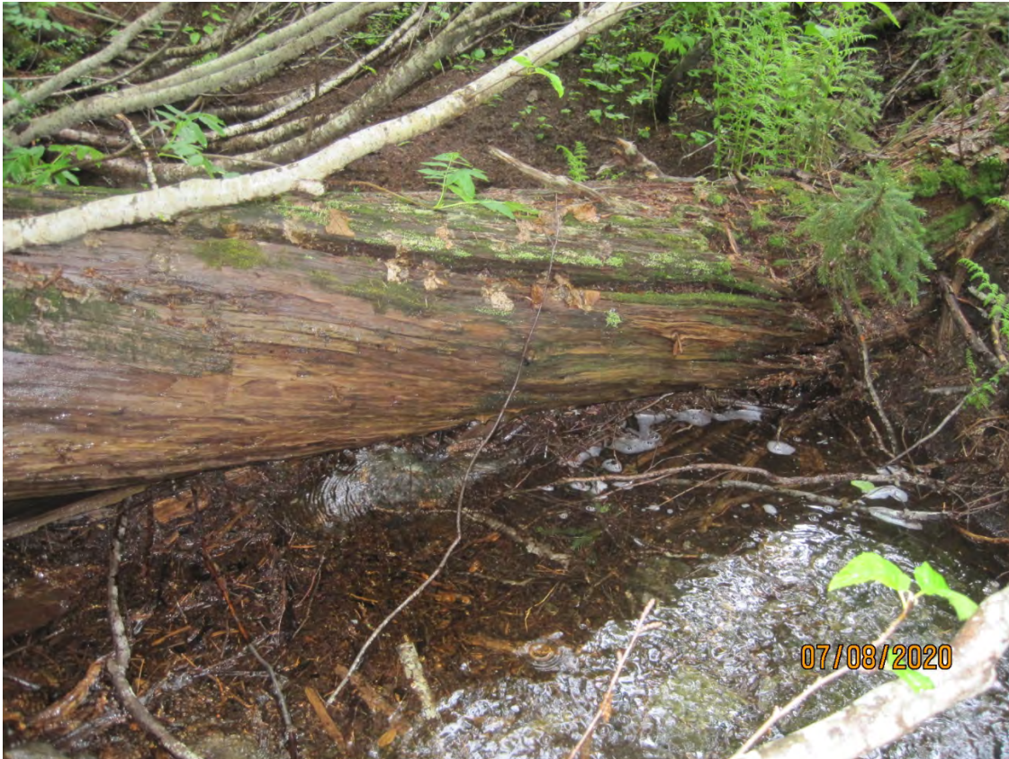
Station 64+37 Perennial stream culvert inlet buried, washout risk
