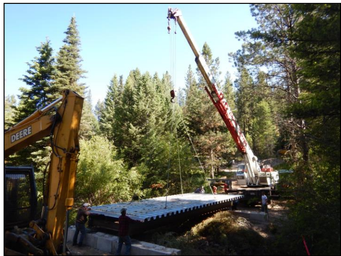
Figure 10 - Road improvements on the Threemile 2 Timber Sale included replacing an old wooden bridge across Spring Gulch with a steel bridge. Photo Credit: J. Parke
